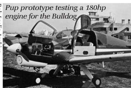
Pup prototype testing a 180hp engine for the Bulldog
